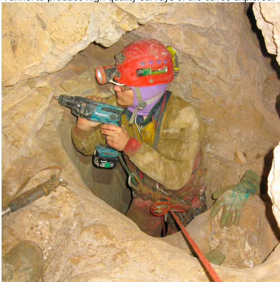
Above: Using a rotary-hammer drill to place an anchor in the rock above an un-descended shaft.
